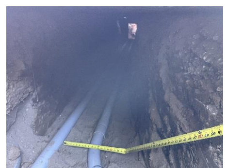
Trenching power at Muir Beach site with Muir Beach Fire.
