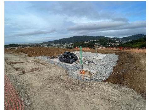
Construction progress at Skyview.
